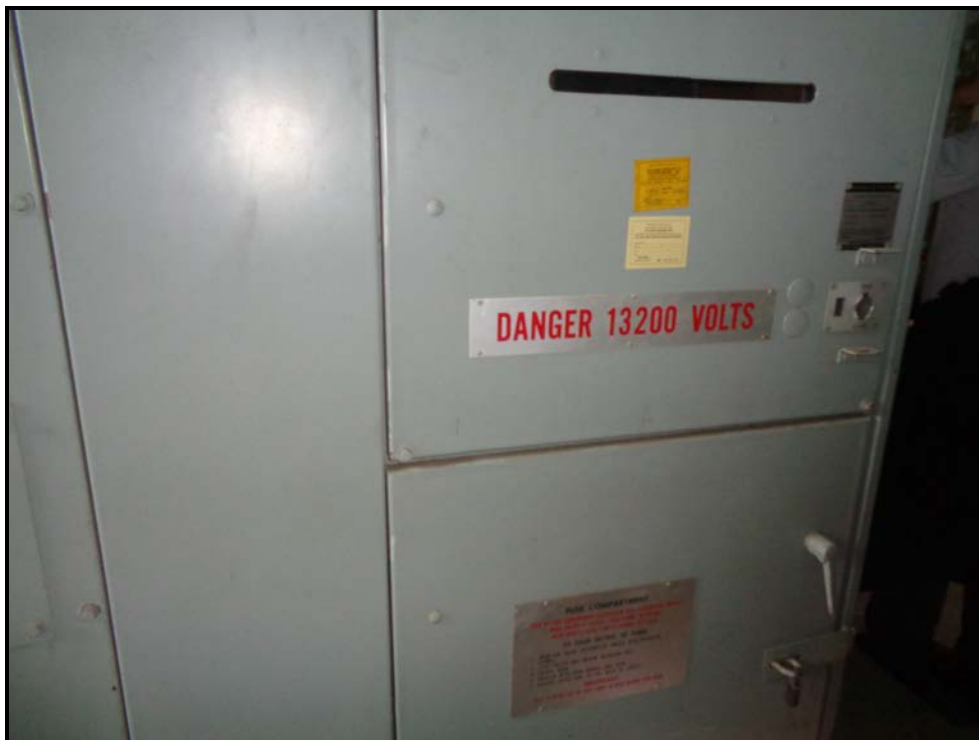
Photograph 10: View of a transformer located in the boiler room of the basement.
