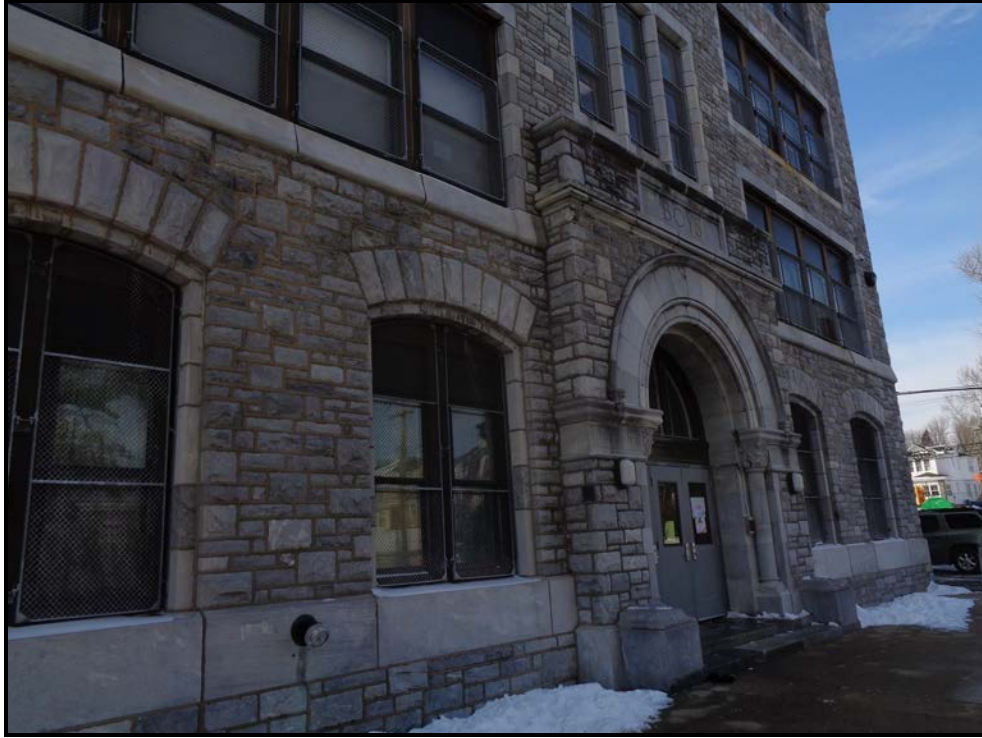
Photograph 3: View of a portion of the school's eastern façade.
