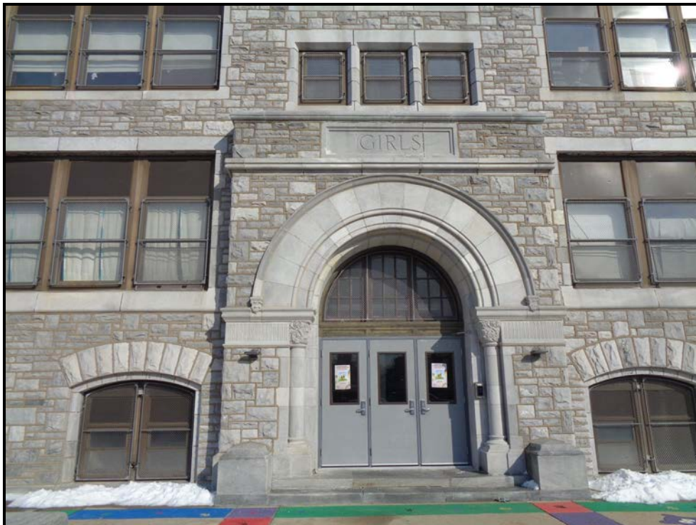
Photograph 2: View of a portion of the school's western façade.
