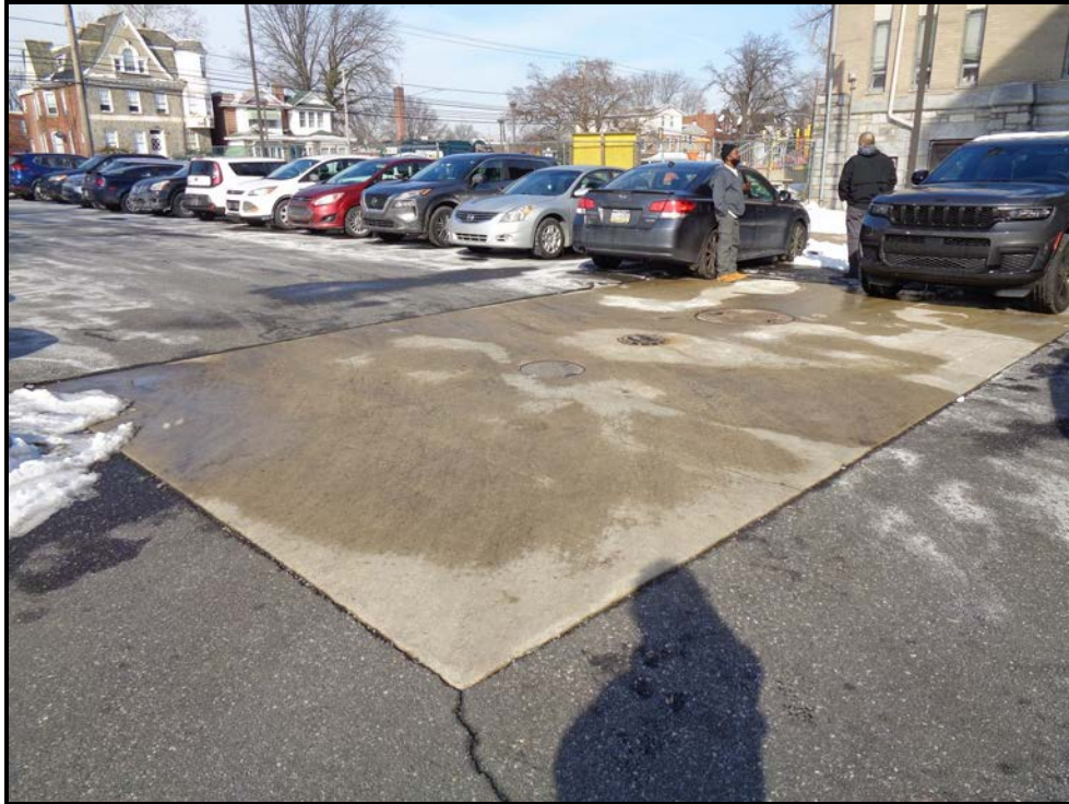
Photograph 7: View of concrete pavement within the properties western parking lot containing an underground storage tank (UST).
