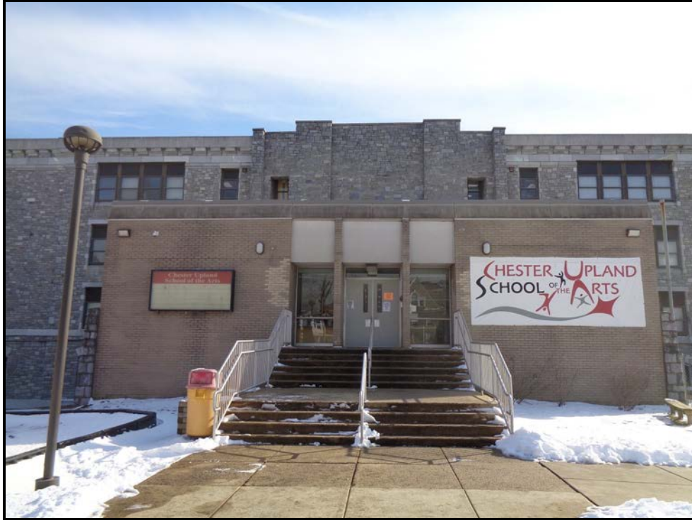
Photograph 1: View of the school's northern facade.
