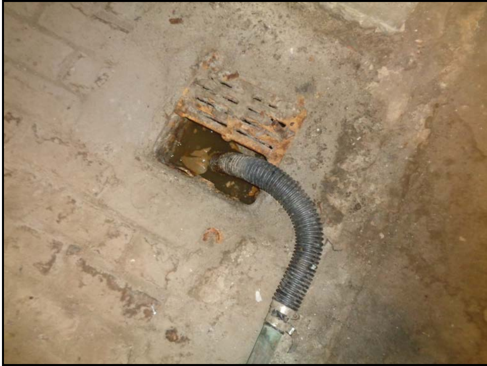
Photograph 11: View of a floor drain located in the basement of the structure .
