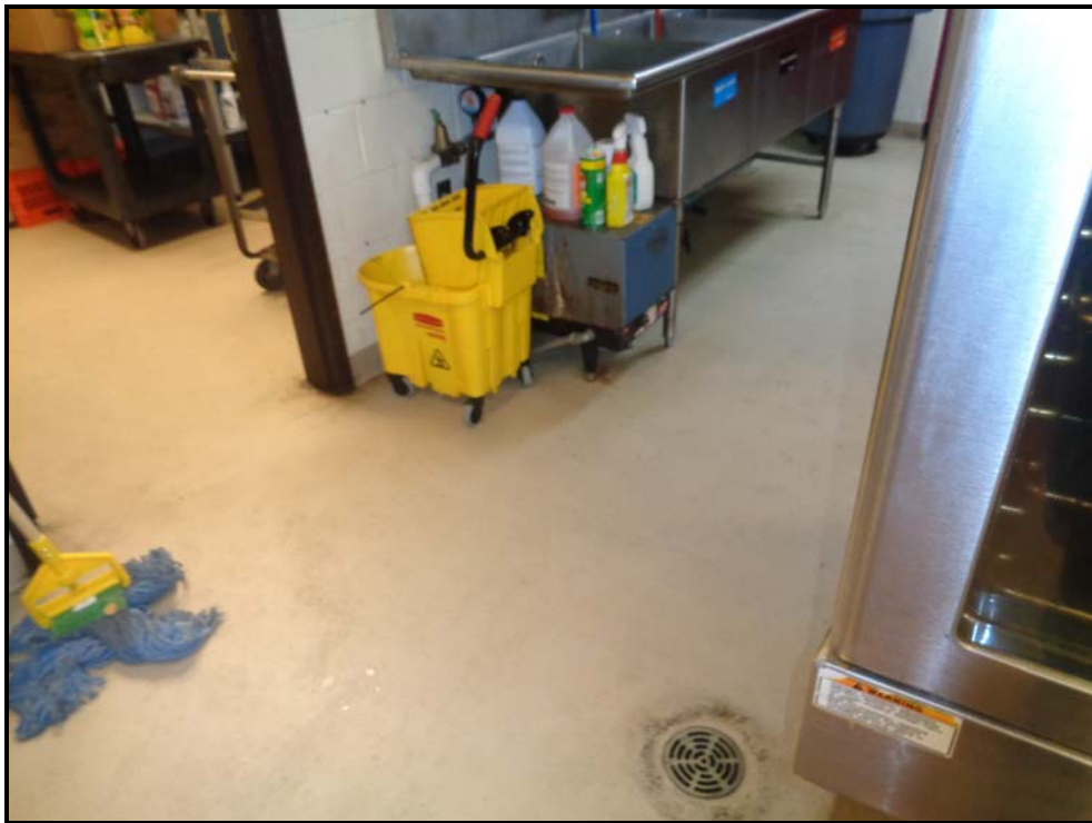
Photograph 12: View of a floor drain located in the school.
