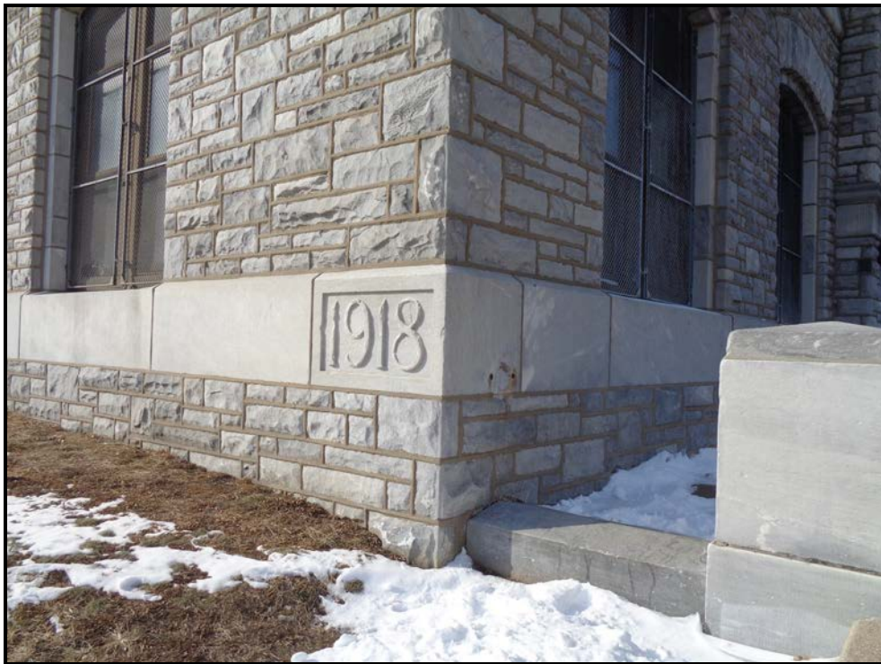
Photograph 4: View of the building's cornerstone.
