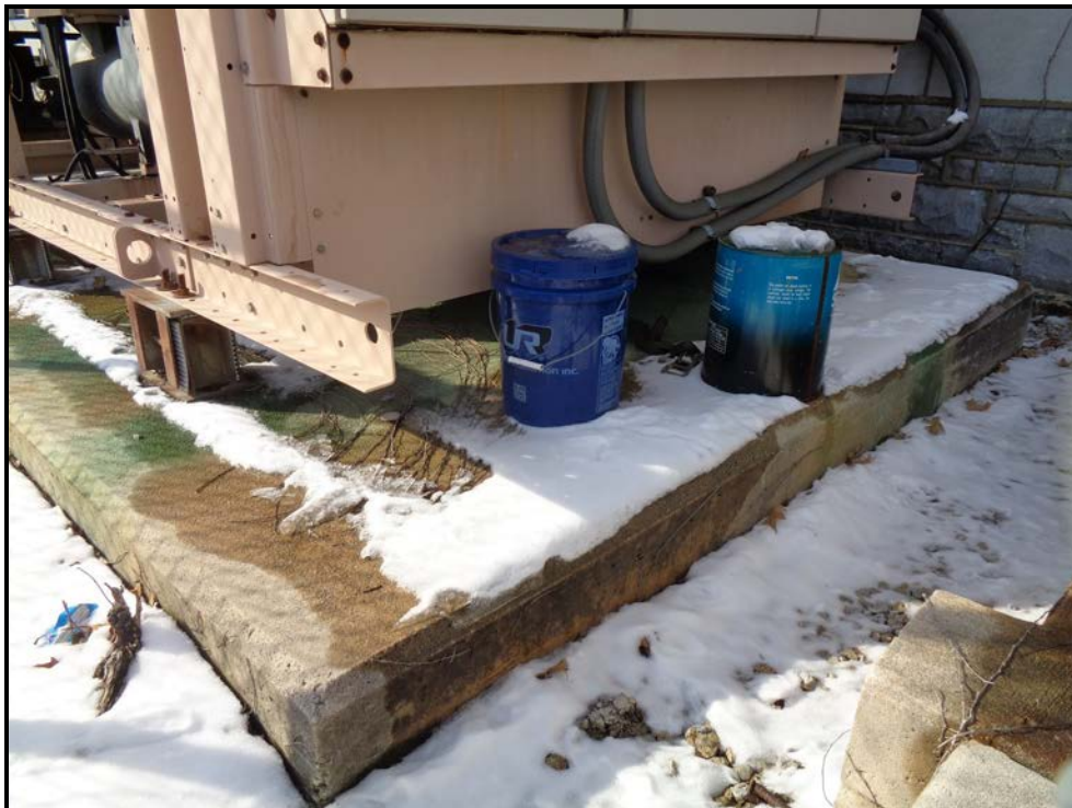
Photograph 6: View of a 5-gallon container of polyol ester compressor oil and a blueish-green colored stained concrete surface, located along to the building's southern façade.
