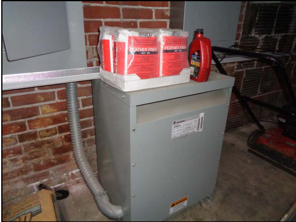
Photograph 9: View of a transformer located in the fan room of the basement.
