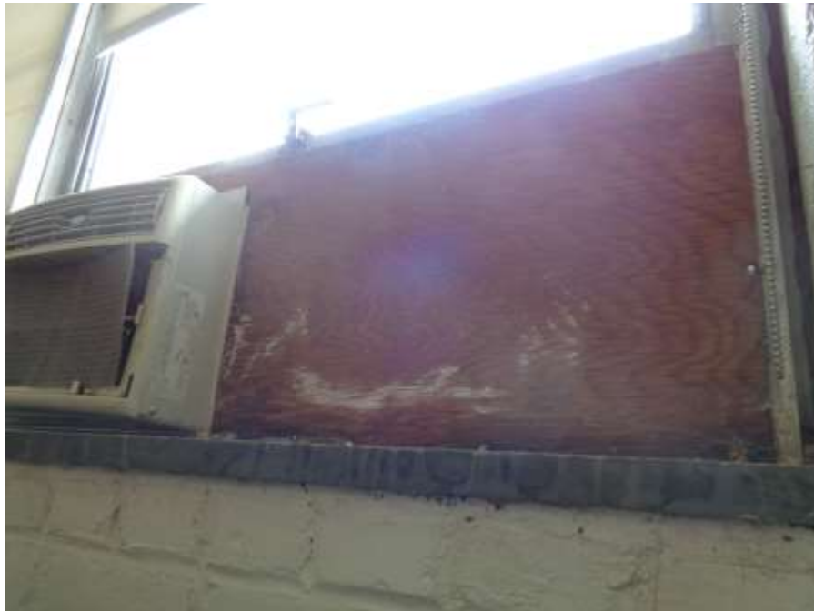
Photograph 6: Wood window spacer with AC unit in Room 14.
