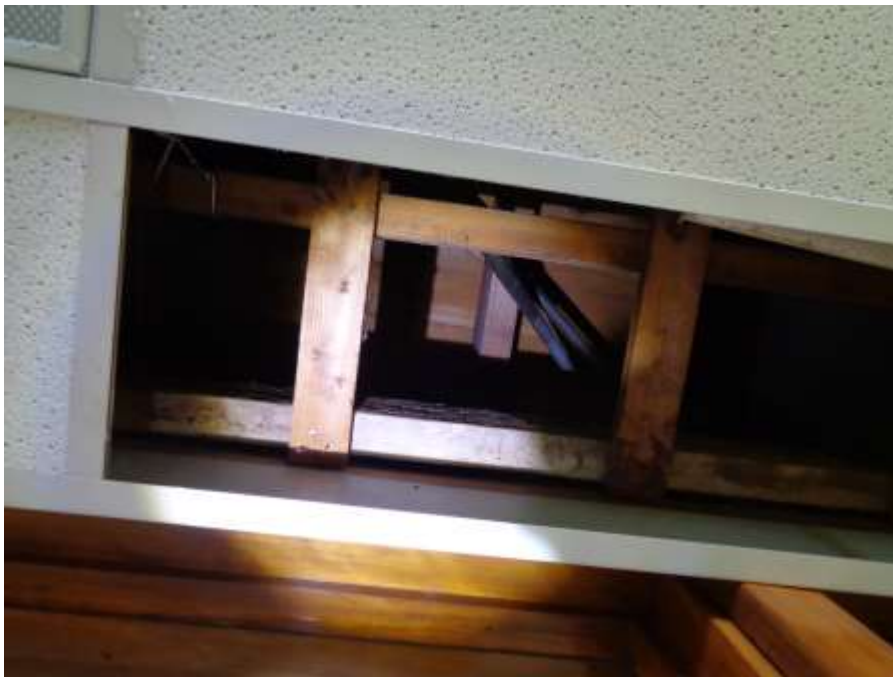
Photograph 4: Wood framing located above the ceiling.
