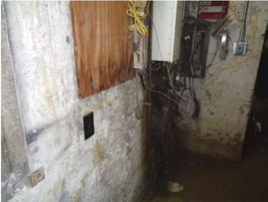
Photograph 5: Wood wall mount with visible mold growth.
