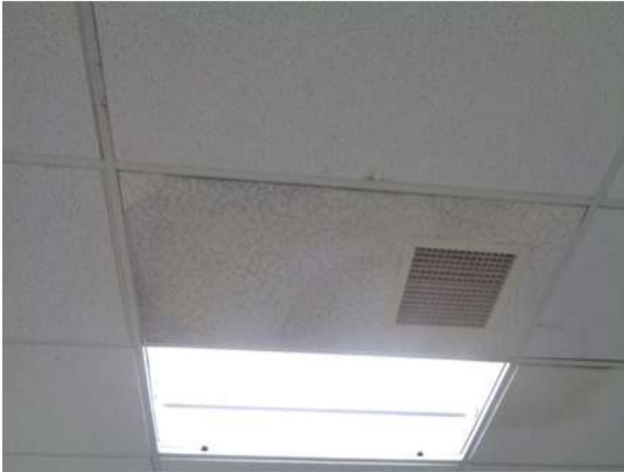
Photograph 3: Examples of stained ceiling tiles observed throughout.
