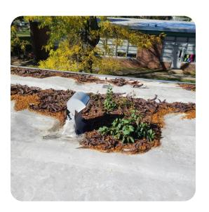
Plants are growing out of debris in the roof. Debris is clogging drains.
