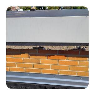
Rebar in exposed concrete is rusting casing the concrete to spall. Building sealants are failing.
