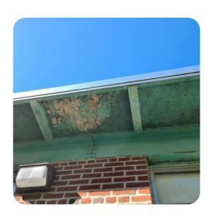
Wooden soffits are starting to rot. Exposed steal beam is rusting.
