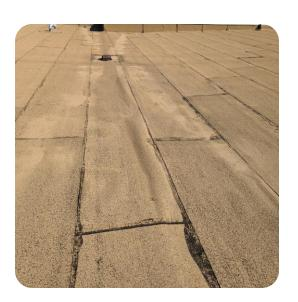
Blisters in cap sheet. Chimney masonry and sealants are failing.
