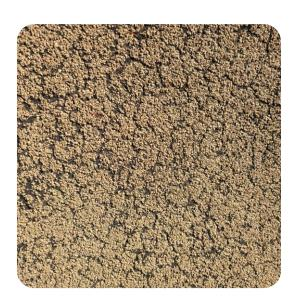
Most of granules have worn off the cap sheet, causing the asphalt to oxidize. Scrim is exposed in deteriorated cap sheet.
