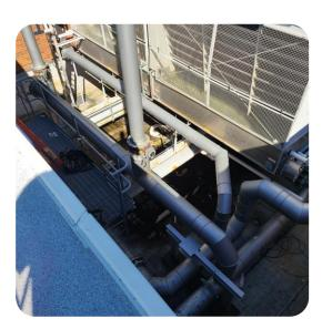
Open hood vent. Cooling tower on Roof 3 is spilling large amounts of water on the roof creating ponding water. Jobsite materials should be properly stored on the roof to not puncture the membrane. Granule loss.
