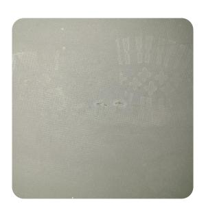
Membrane has deteriorated down to scrim. Punctures in roof.
