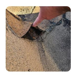
Open seams. Improper flashing detail.
