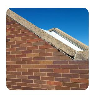
Stone copings are spalling. Window sealants are failing. Boards with nails need to be store properly on the roof to not puncture the roof membrane.
