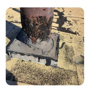
Alligatoring membrane. Scrim is exposed . Open pitch pockets. Granule loss.
