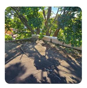
Plants are growing in debris on the roof. Debris is clogging roof drains.
