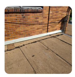
Previous repairs to seams and flashings. Low flashing heights will have to be raised if the roof is replaced.
